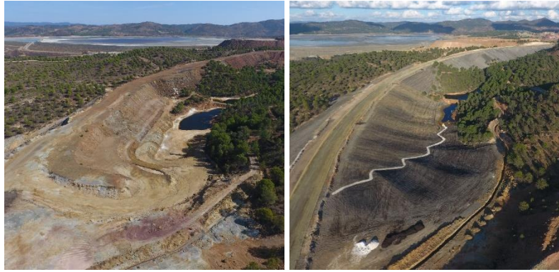
Figure 2. Geomorphic Restoration of a sector of the Riotinto mine (Atalaya Mining, Huelva, Spain). Left, pre-restoration scenario in 2021. Right, post-restoration result, in 2024 (photo by Atalaya Mining).
