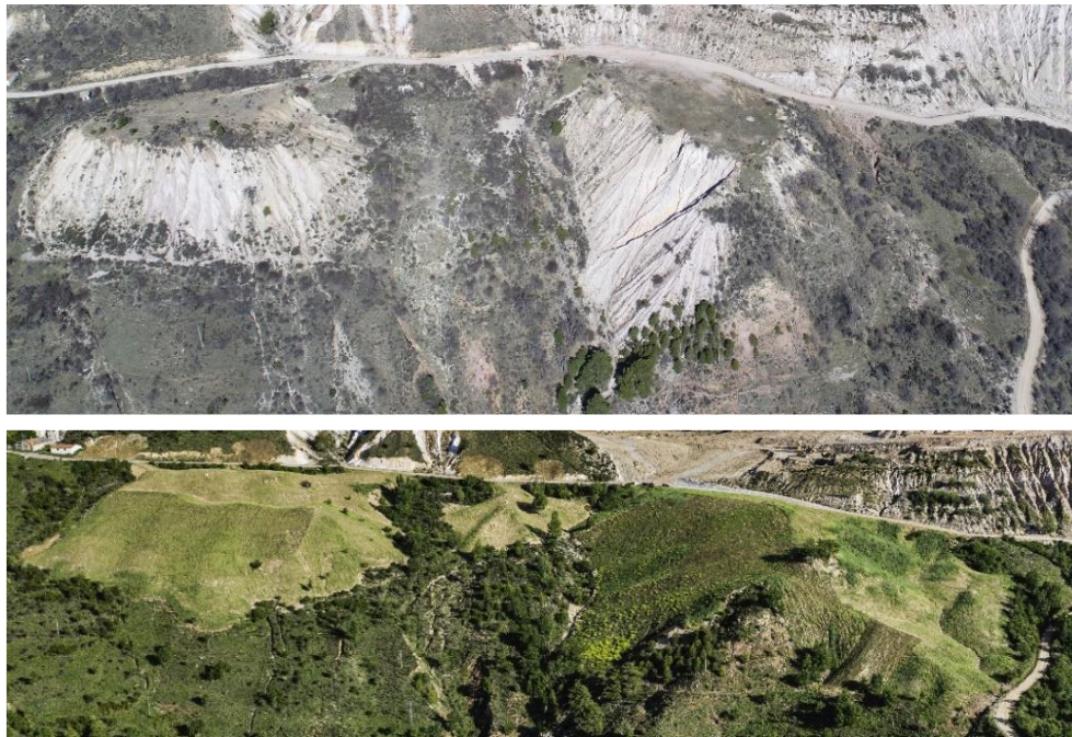
Figure 1. Geomorphic Restoration of the external waste rock dumps of the Santa Engracia mine (Peñalén, Guadalajara, Spain), carried out with the GeoFluv – Natural Regrade method. Left, pre-restoration situation, March of 2020 (photo by Diedro). Right, post-restoration situation, May of 2021 (photo by M.A. Langa).
