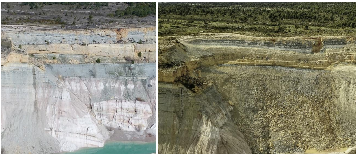
Figure 3. Geomorphic restoration of the former highwall of the Santa Engracia mine (Peñalén, Guadalajara), carried out following the Talus Royal method. Left, pre-restoration condition, in 2020 (photo by Diedro). Right, post-restoration situation, in 2024 (photo by M.A. Langa).
