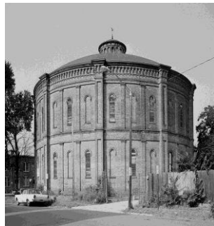
Figura 2.2. Gasómetro de la Troy Gas Light Company (Rensselaer County, New York).
