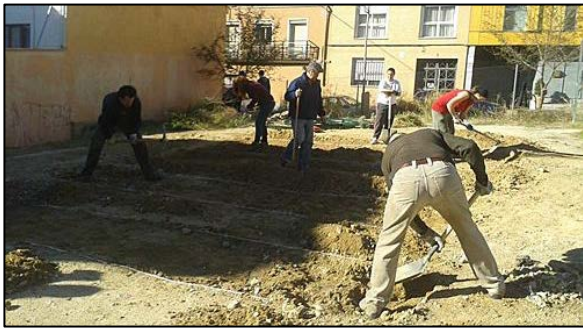
Figure 5. Building the site, February 2014
