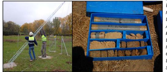
Fig. 3. (a) Left: Uprising of the meteorological tower. (b) Right: A set of core rocks. Note that the first 1.5 meters are encased in PVC to preserve the soil structure and composition.
